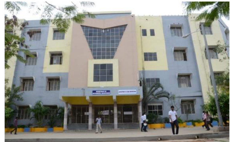
Civil, Mechanical and Mining Engineering Block
