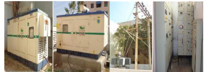
❖ Electrical Power: 3 generators of capacity 62.5 KVA, 125 KVA, 250 KVA and 400 KVA transformer
